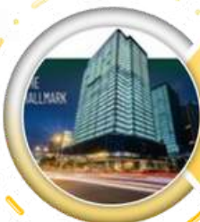
HALLMARK BUILDING - FLOOR 15& 19
